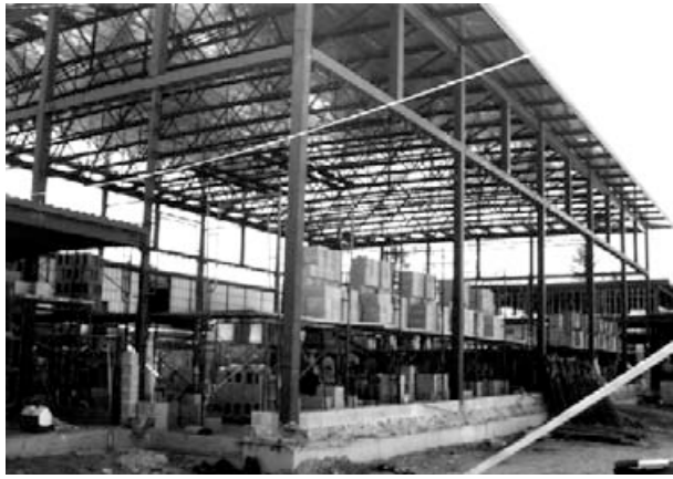
The CMU masonry is loaded on the scaffolding and prepared for installation at the two-story addition at the Coolidge Middle School. This area houses the Theatre and Laboratory Facilities as well as the Media Room and Library.
