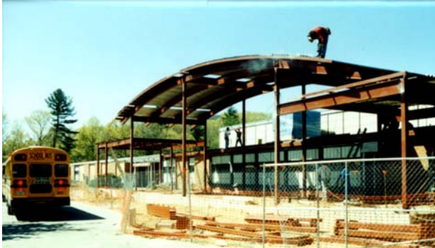
View of the new, steel framed barrel roof at the addition to the front of the school under construction.
